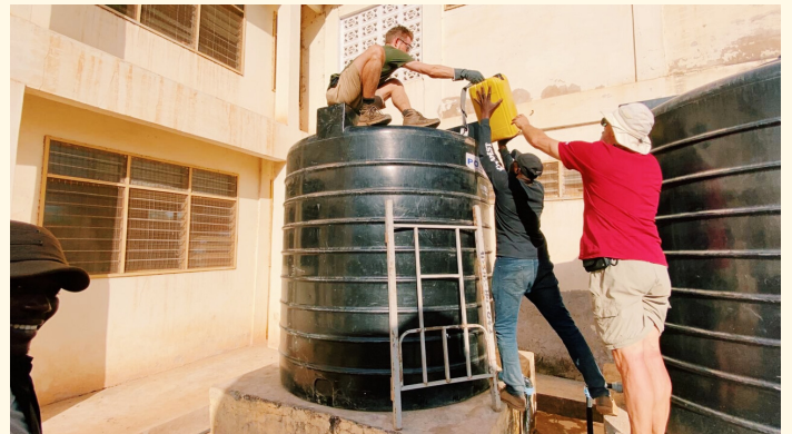
Schock chlorinating the polytanks at the girls dorm.
