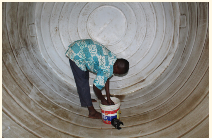
Cleaning out water storage tanks.
