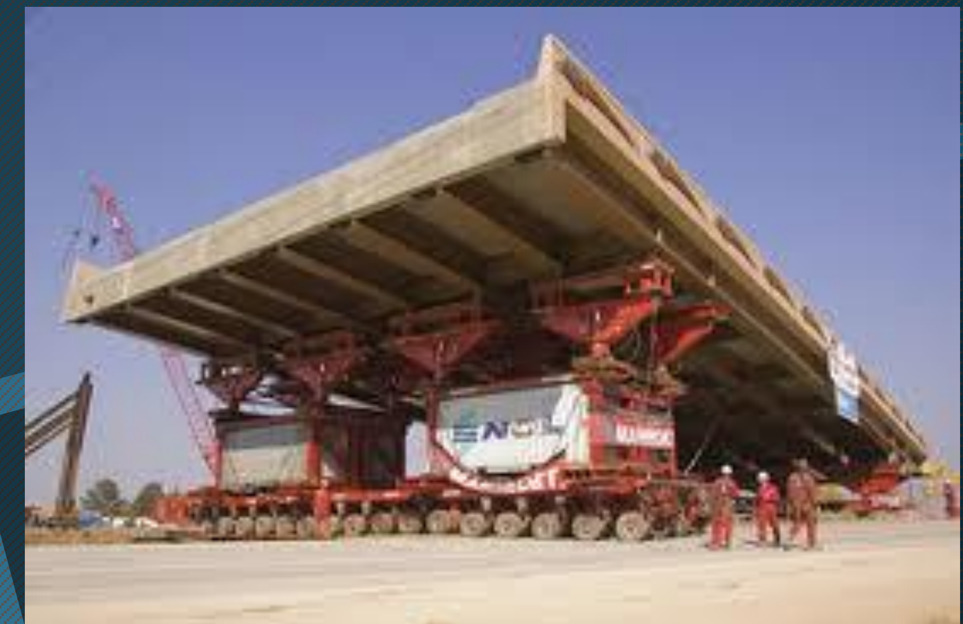
Utah DOT using CM/GC to perform accelerated bridge construction.
