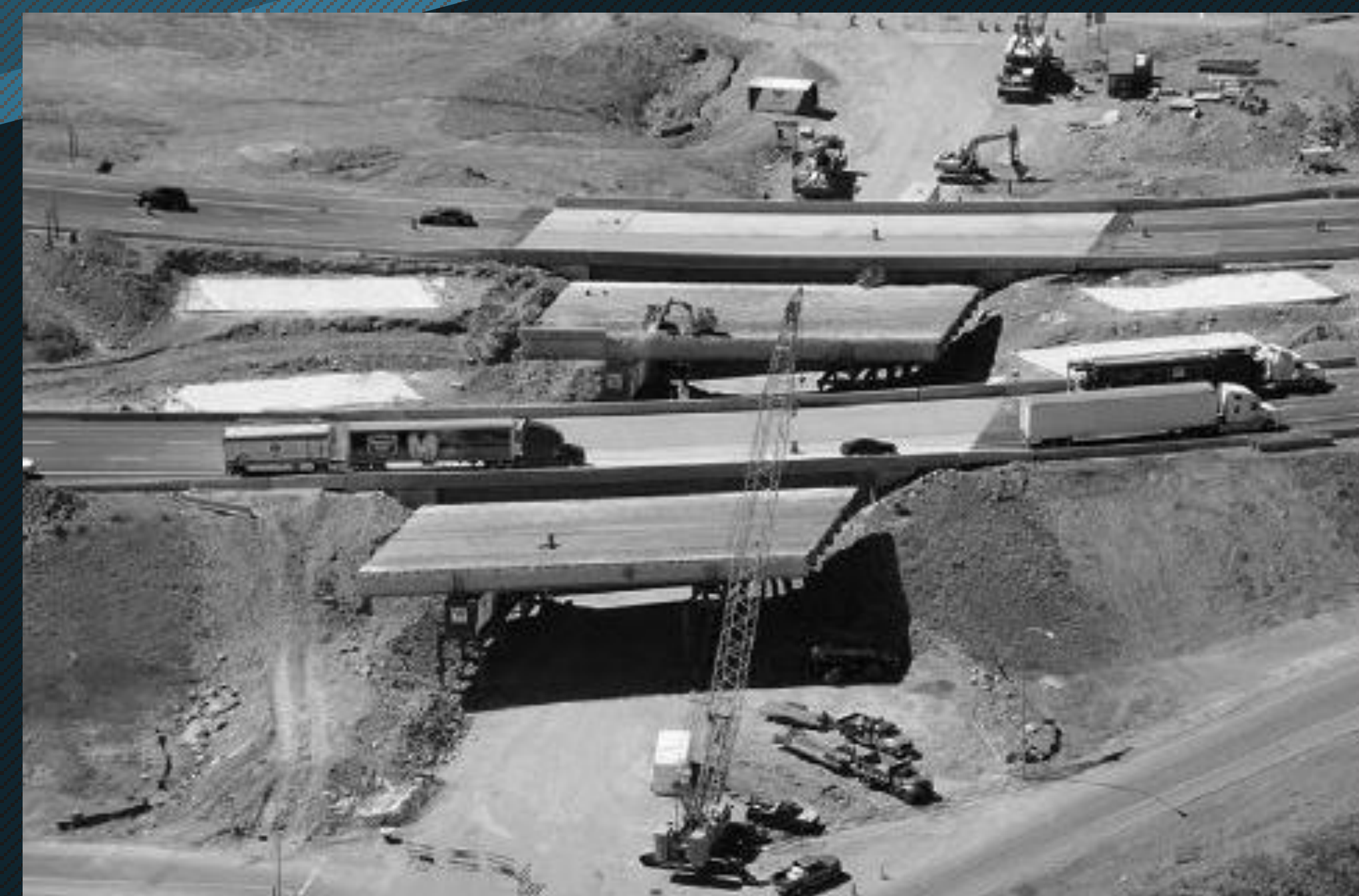
Utah DOT using CM/GC to perform accelerated bridge construction.
